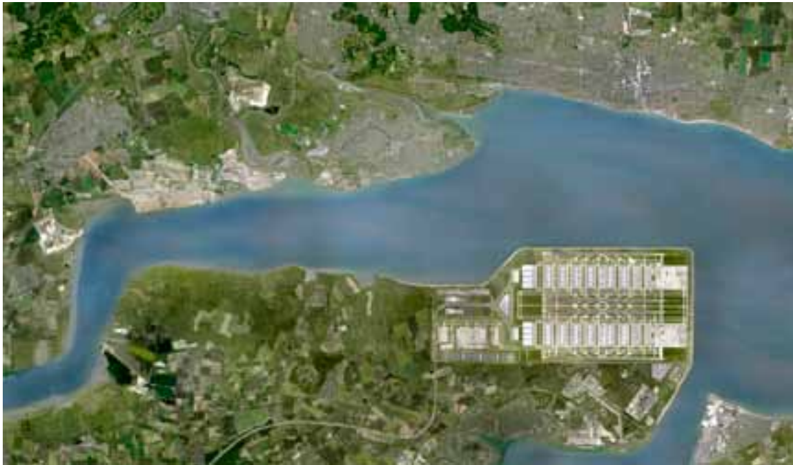
BELOW Aerial view of the Thames Hub Airport, with runways laid out to minimise the impact of noise
